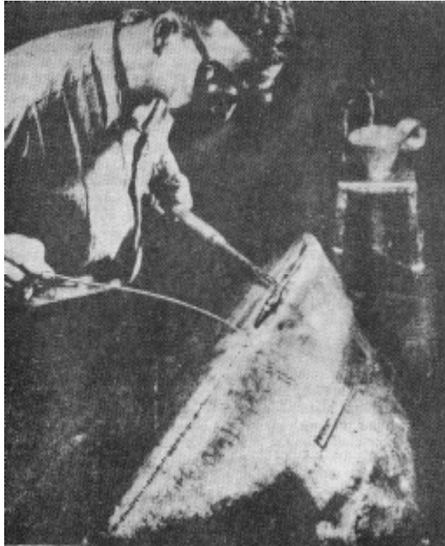
Fig.5.12. Torch Welding a Magnesium Aircraft Oil Tank
