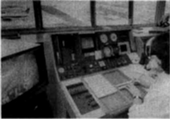
Plate 9 In the Manchester Airport visual control room. On the left of the CCTV information display may be seen the D/F readout. To the right are the wind vane and anemometer dials and the radar distance-from-threshold indicator (DFTI). The buttons control the R/T channel in use or private wire telephone circuit. The controller is updating a flight progress strip. The display on the left is that of the Racal AR18x Airfield Surface Movement Indicator. (Photo: Racal )
