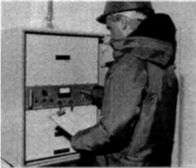
Plate 18 The Racal RDB100B watt non-directional beacon. Two transmitters are included, one of which is in standby mode but automatically takes over service in the event of main equipment failure.
