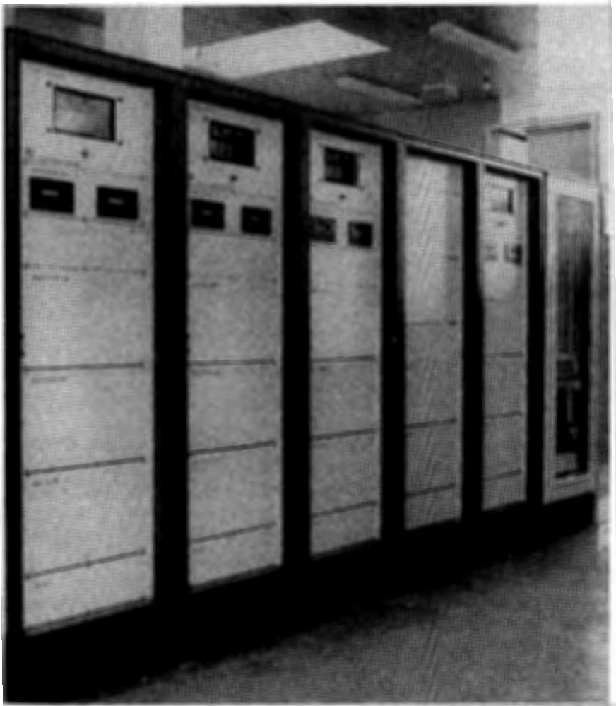
Plate 48 Hindsight recorders. The local control unit is at the top of each rack below which is the Mass Storage Unit; System Control Unit; data interface unit. (Photo: Walton Radar Systems)
