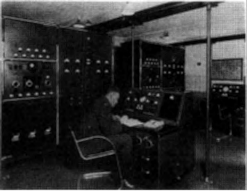
Plate 5 The transmitter room of a Chain Home (CH) radar station. (Photo Marconi)
