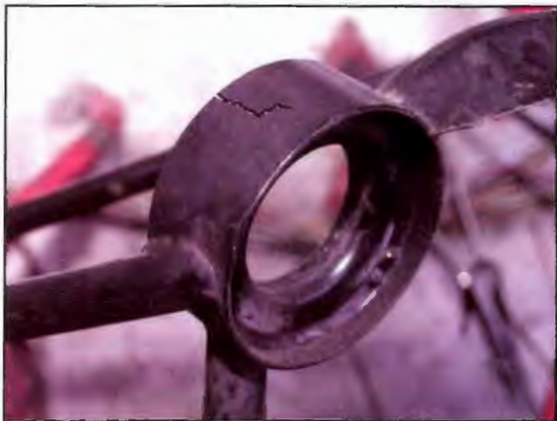
Figure 13-18. Examine the engine mount for cracks. If cracks are suspected, use at least a 10-power magnifying glass to perform a more thorough inspection. In some cases, it may be necessary to remove the paint from the mount to perform a dye penetrant inspection.
