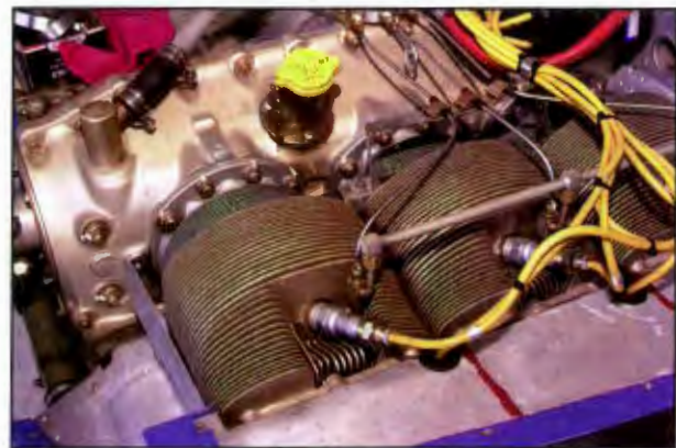
Figure 14-8. Improperly secured fuel injector lines could cause the soldered ends to fracture and leak.
