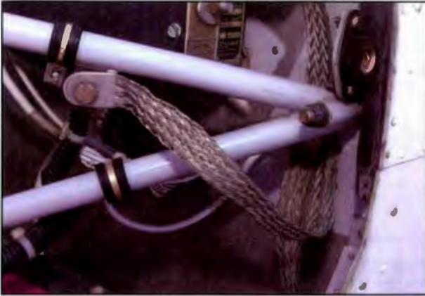
Figure 14-4. A common fault affecting powerplant electrical systems is a defective ground circuit. Always check that ground wires are properly secured and free of corrosion. Also, verify that any bonding cables or straps are in place and properly attached between the engine and airframe.
