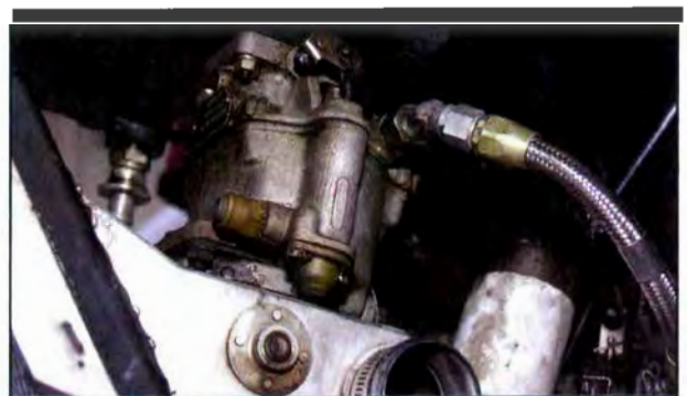
Figure 14-7. Fuel stains may indicate a leak from a worn accelerator pump seal.
