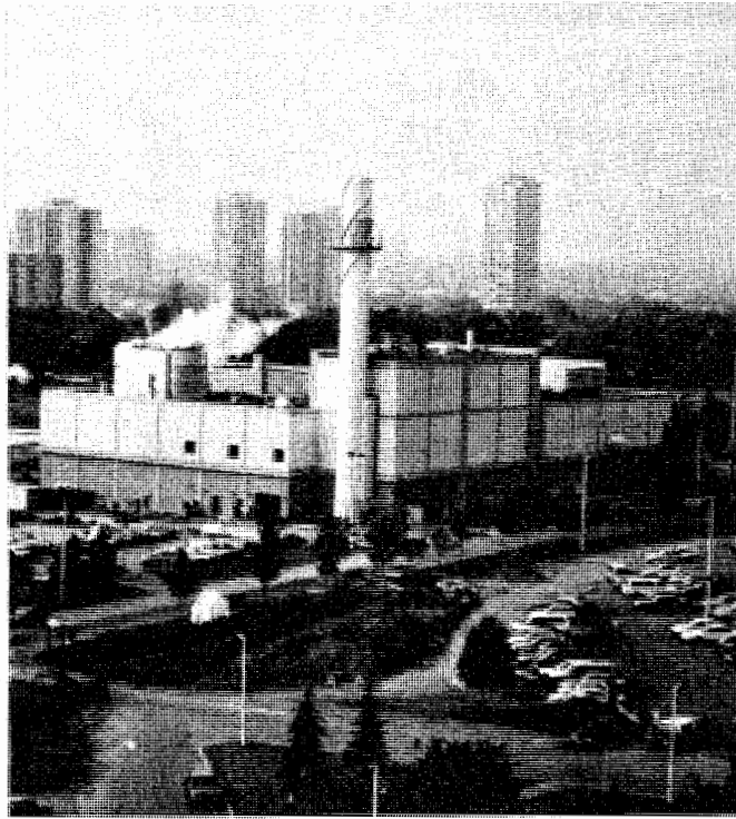
FIG. 1.19 70 MW combined cycle plant [courtesy Stewart and Stevenson]
