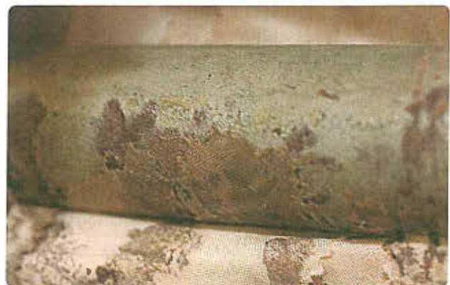
Figure 18-5. Rust on structural components.
