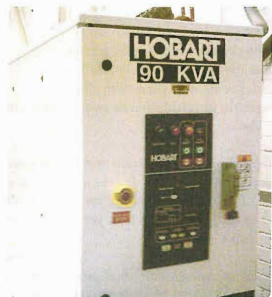
Figure 17-22. A stationary electrical power unit.
