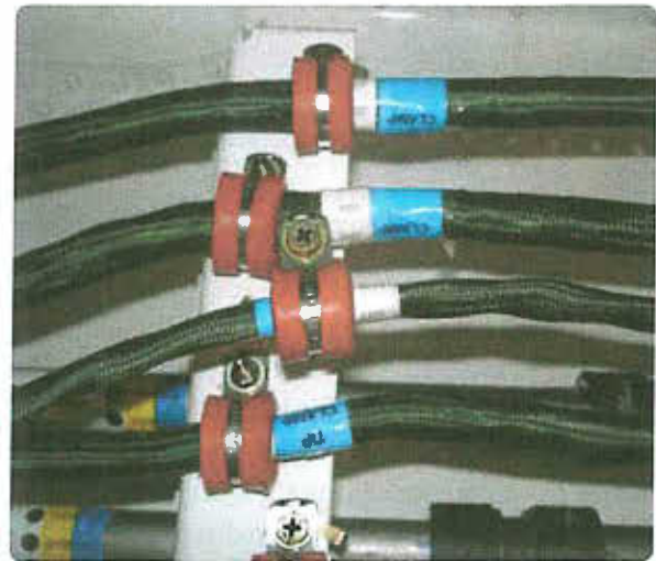
Figure 7-35. Positive separation of wires and wire clamps.
