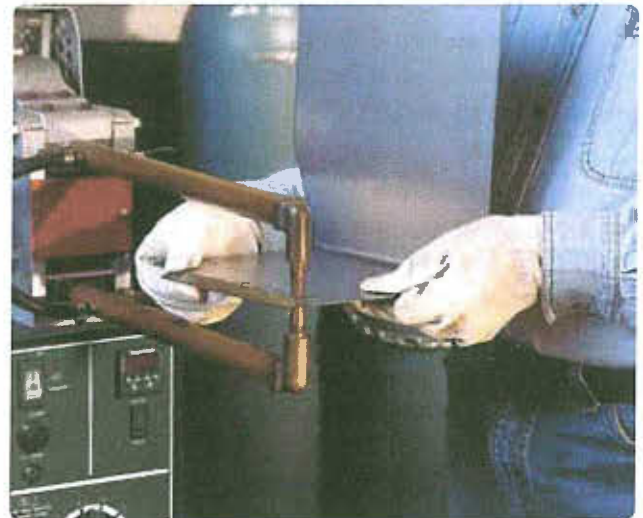
Figure 15-11. Spot welding thin sheet metal.
