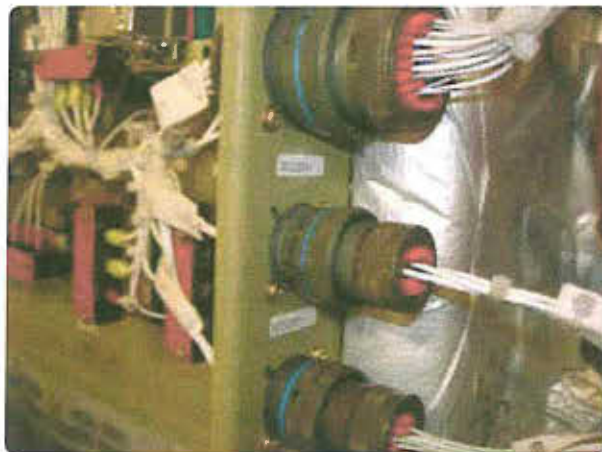
Figure 7-21. Connector arrangement to avoid wrong connection.
