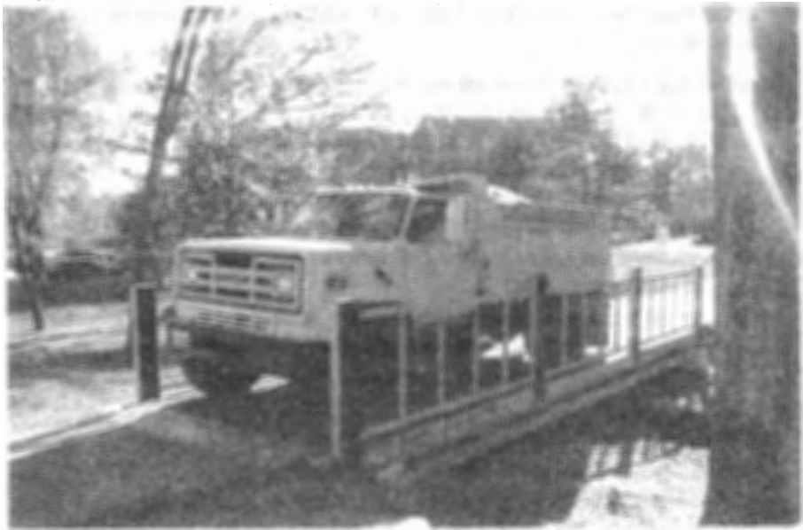
Figure 1-5. The composite bridge installed at the UMR campus with a truck on it.
