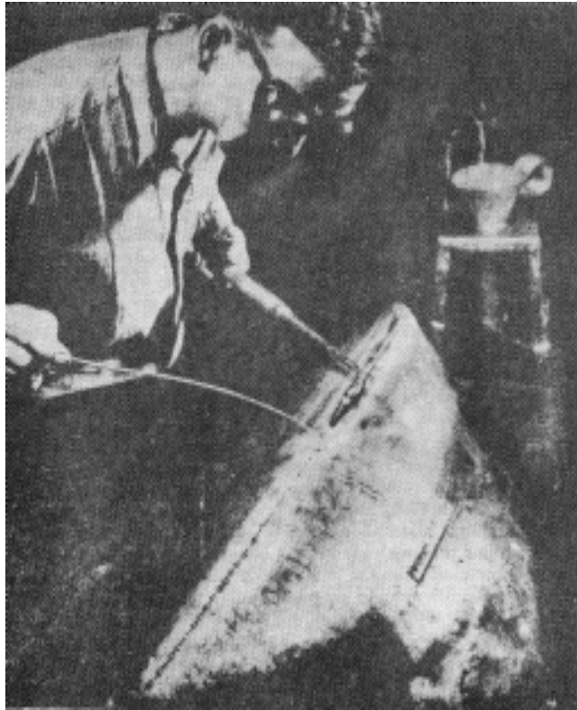
Fig.8.12. Torch Welding a Magnesium Aircraft Oil Tank
