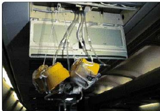
A passenger service unit (psu) is hinged over each row of seats in an airliner. Four yellow continuous flow oxygen masks are shown deployed. They are normally stored behind a separate hinged panel that opens to allow the masks to fall from the PSU for use.
