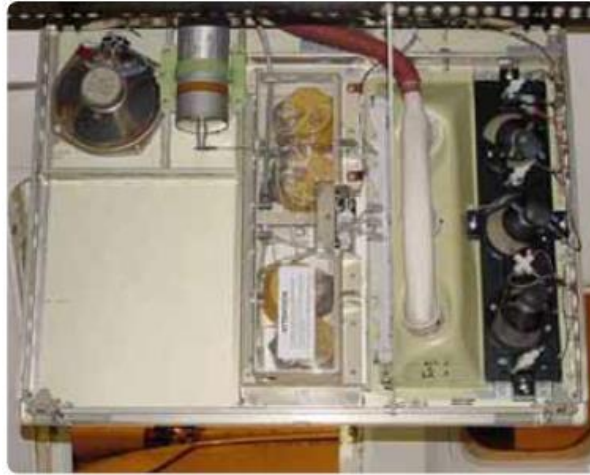
An oxygen generator mounted in place in an overhead passenger service unit of an air transport category aircraft.
